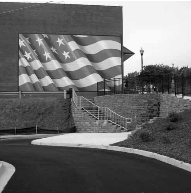
A new staircase, flag mural and landscaping (bottom) have transformed the area adjacent the TheatreWorks building.
